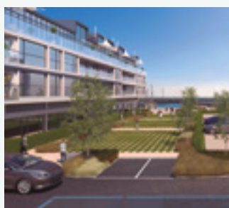
Marina Village Greystones. 205 stanova i 153 kuće. Irska. Aquarea
